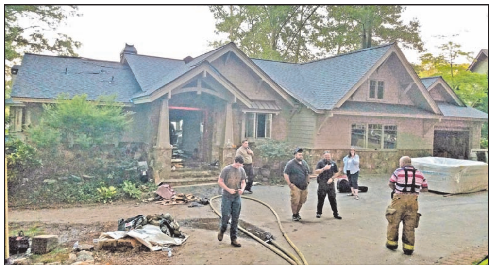
The home experienced shingle damage, along with more extensive damage to some of the interior of the home. Photo/Towns County Fire & Rescue
